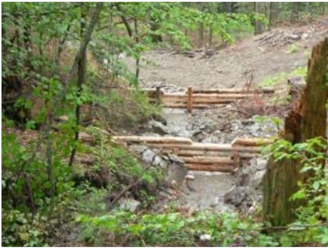
Log dams cascade repairing an erosion gully.
