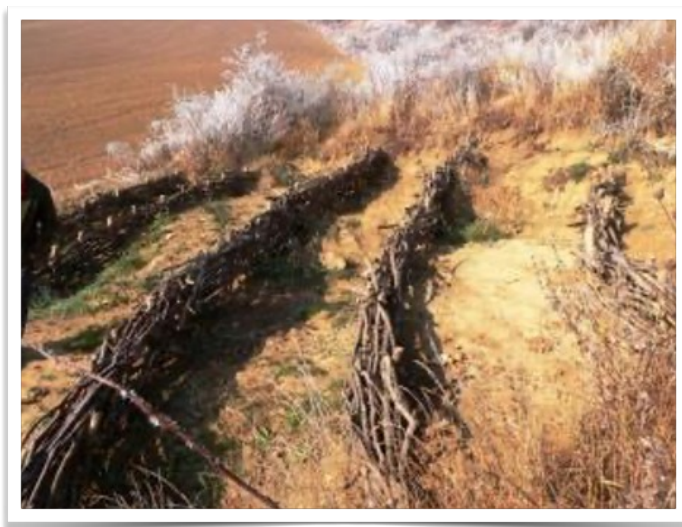
Cascade of small barrier dams. Sustainable solutions, using local by-product branches.
