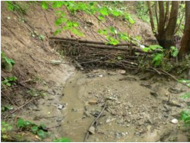
Check dams preventing erosion.
