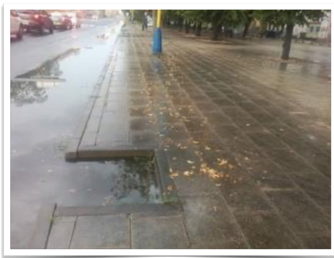
Left: Stormwater runoff is treated as a nuisance in Košice city, drained out to the nearest river, polluting it, and leaving the city dry during rainless periods. Picture shows that the tree roots cannot access moisture, while during rain, puddles collect on the road. Right: Roads in Košice city flood after heavy rains. Impervious paved roads give the rainwater no room to seep into the ground and nourish the vegetation. Urban bioretention methods would slow the rainwater down and prevent floods.
