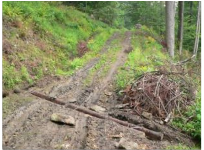
Sustainable road channel drainage adjacent to the logging road.
