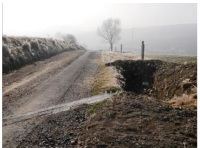
Intercepting cross dip and cross drain. Road drainage, utilizing a slope gradient.
