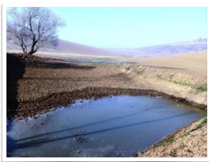
Bioretention pond after the rainfall.
