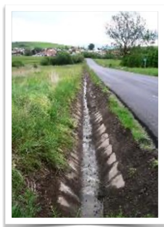
Photo on the left: Inadequate rainwater management drains runoff out and away from the Kavečany town. Middle: Olšava flood, 2010. Right: Flawed rainwater management at Spiš.
