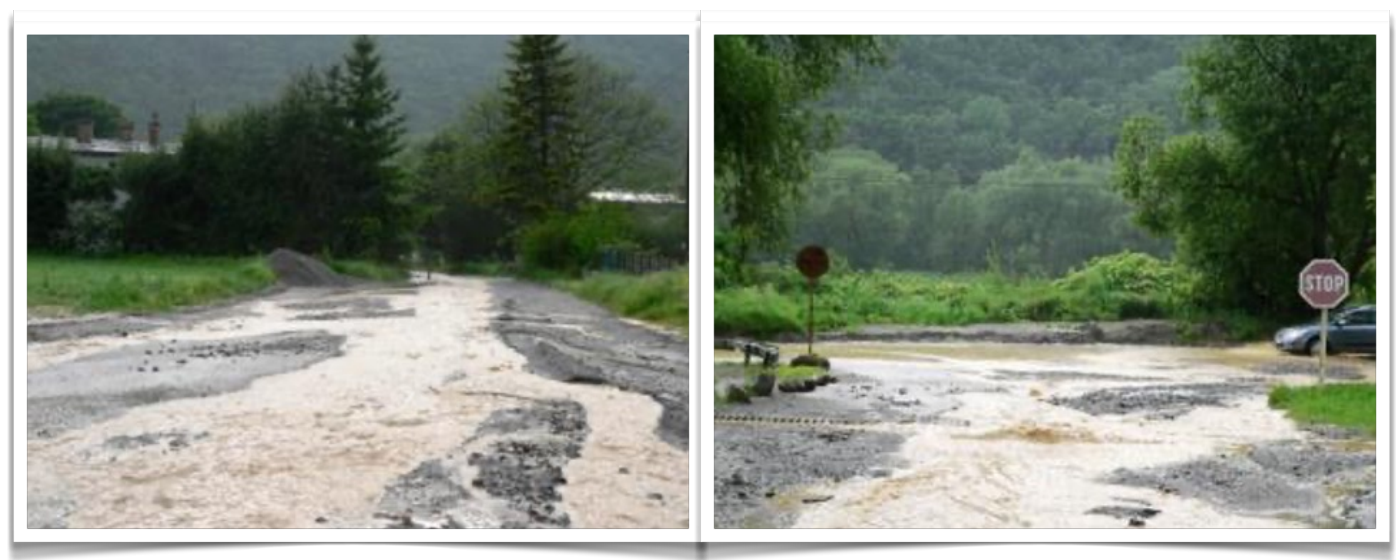
Erosion and land degradation. Regular roads give way to fast-flowing streams amid torrential rains. Flood and road hazard at Trebejov, 2016
