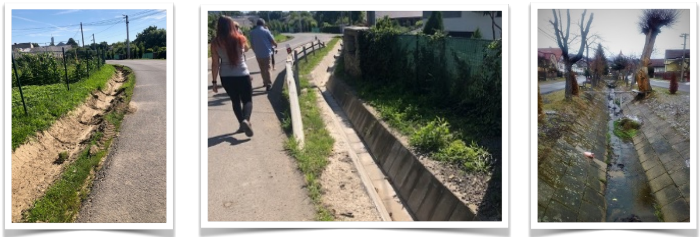
The old water paradigm at Kazimír, Malá Trňa (Třebišov district). The borough is discharging rainwater as an unnecessary resource. Impermeable surfaces seal the soil, reducing water infiltration, further dwindling groundwater supply.
