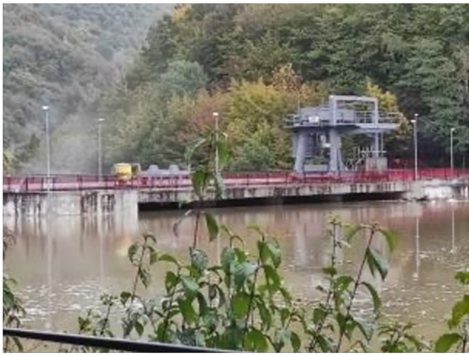
Left: High flood risk level, Ružín dam, October 2020.
