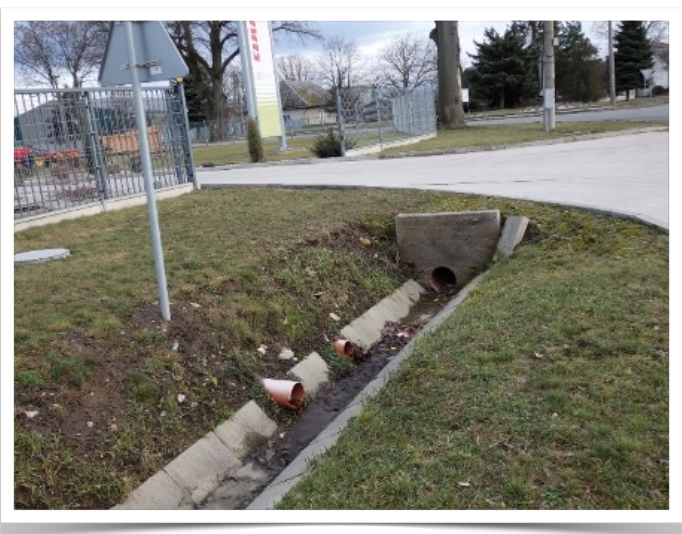
Draining rainwater in the township of Zemplínsky Klečenov (Trebišov). Concrete stream channel. Culvert. Unsustainable channelization and inadequate stream crossings alter hydrology and destroy aquatic life.
