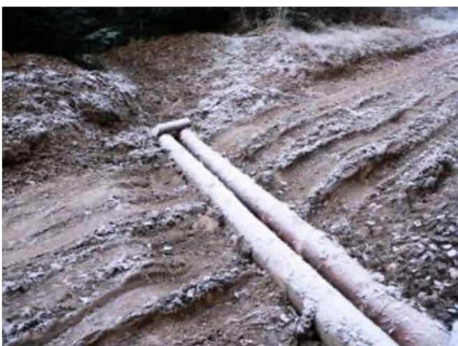
Intercepting cross dip and cross drain. Road drainage, utilizing a slope gradient.
